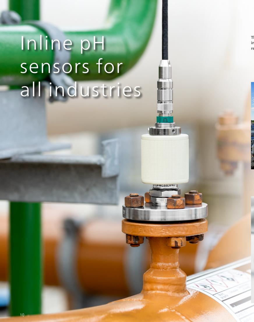
The ProTrode sensors from Metrohm Process Analytics are the perfect solution for a wide range of industrial applications. Our Swiss quality sensors offer type HT and H quality glass, which enable stable readings and accurate measurements over a broad pH range.
